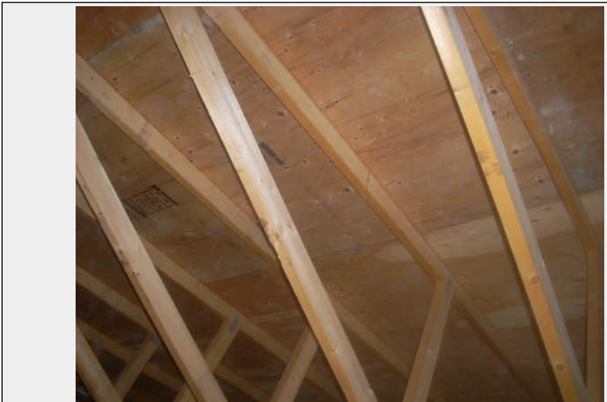
Attic was clean and dry at time of inspection.
